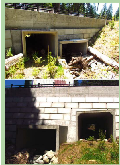
Top: Box culvert wildlife crossing at upstream (North) side of Smiling Creek underneath Princeton Avenue in Northeast Coquitlam; wildlife crossing on the left and the watercourse is on the right.
